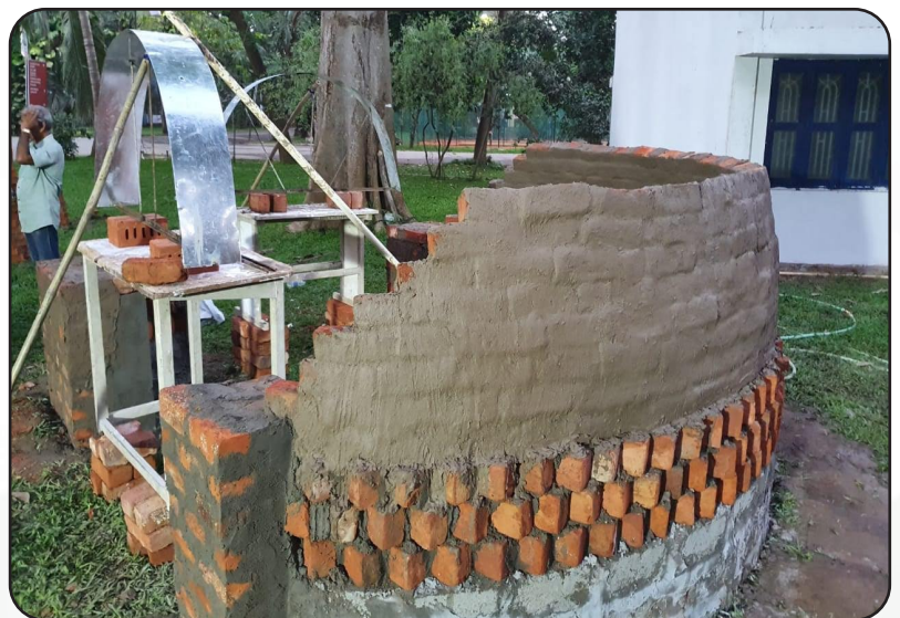
Sustainable Housing – Mud dome construction
